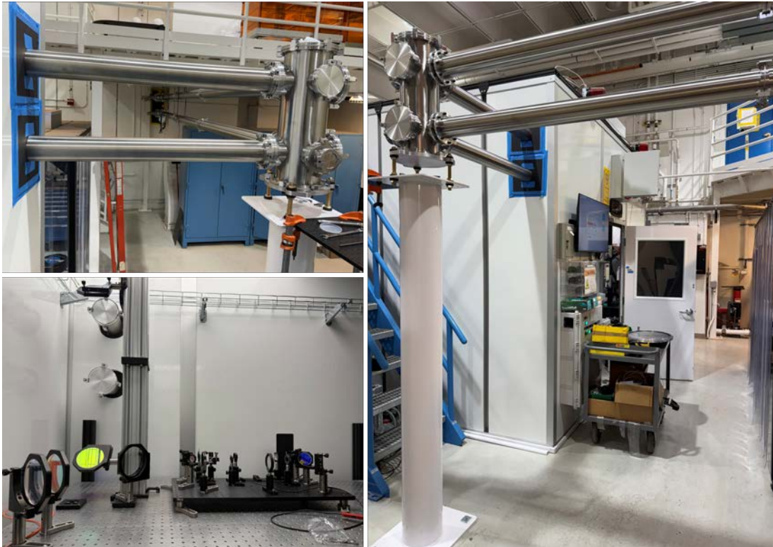
Figure 2-1. (top) Laser beam vacuum transport lines from Z-Backlighter (back wall) to the Mykonos Laser Control Area (left). (right) Beam steering tower. (bottom) Down periscope for beam routing into target chamber and alignment beam injection area and beam diagnostic (bread board).
